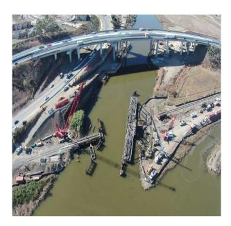
Shimmick Construction is also responsible for the technically challenging replacement of the Haystack Moveable Bridge at the Petaluma River. The current bridge will be replaced with a rolling bascule bridge purchased from Galveston Texas in 2012. In 2014, significant preparation work was undertaken, including:
