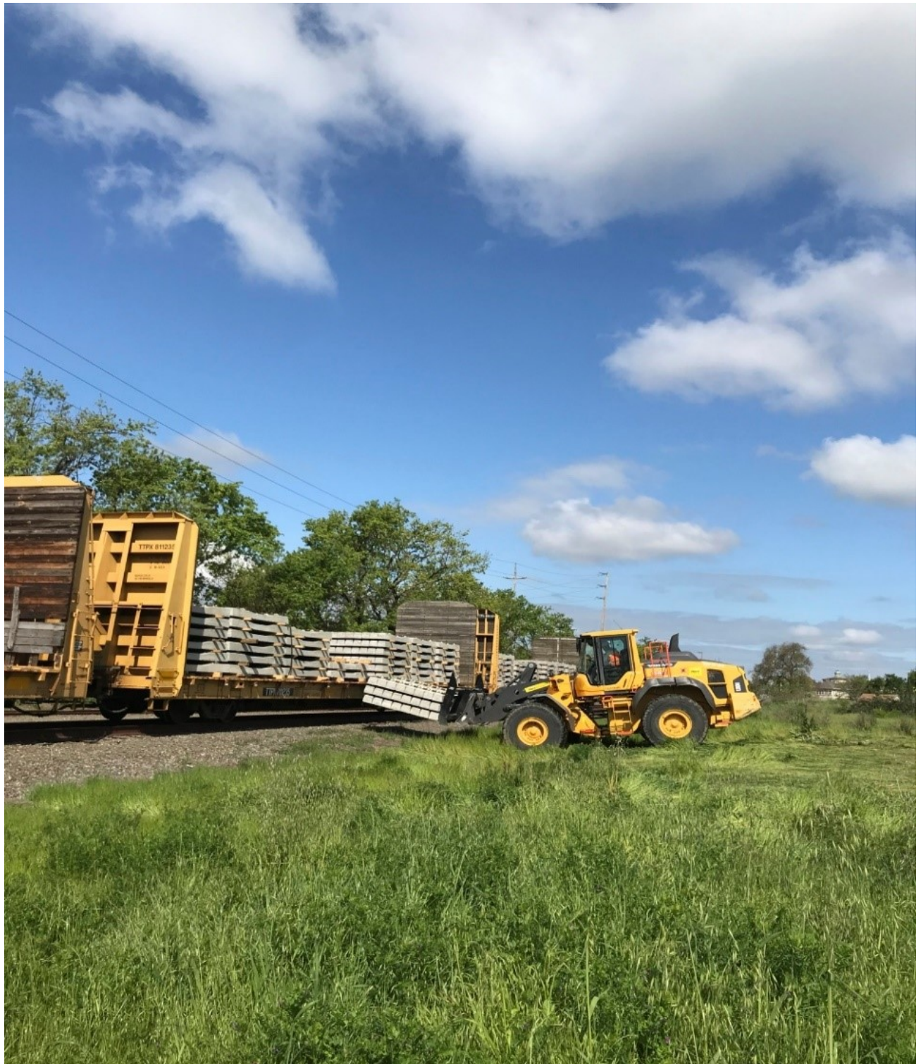
Concrete Tie Delivery
