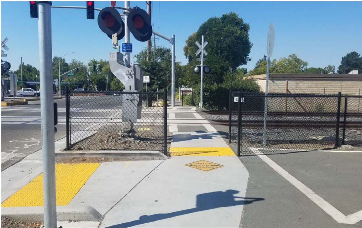
East Cotati Ave., Cotati- Pedestrian Channelization Fence
