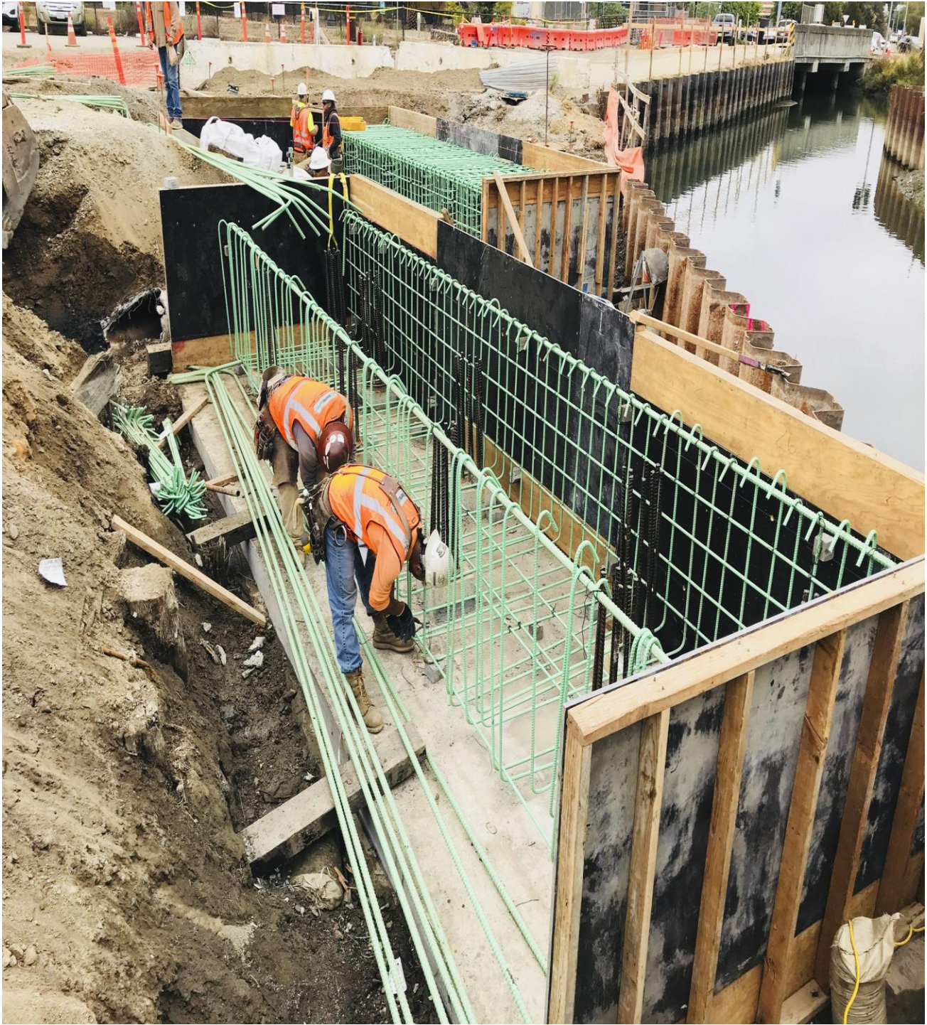
San Rafael Creek Bridge Rebar Installation for the bridge foundation
