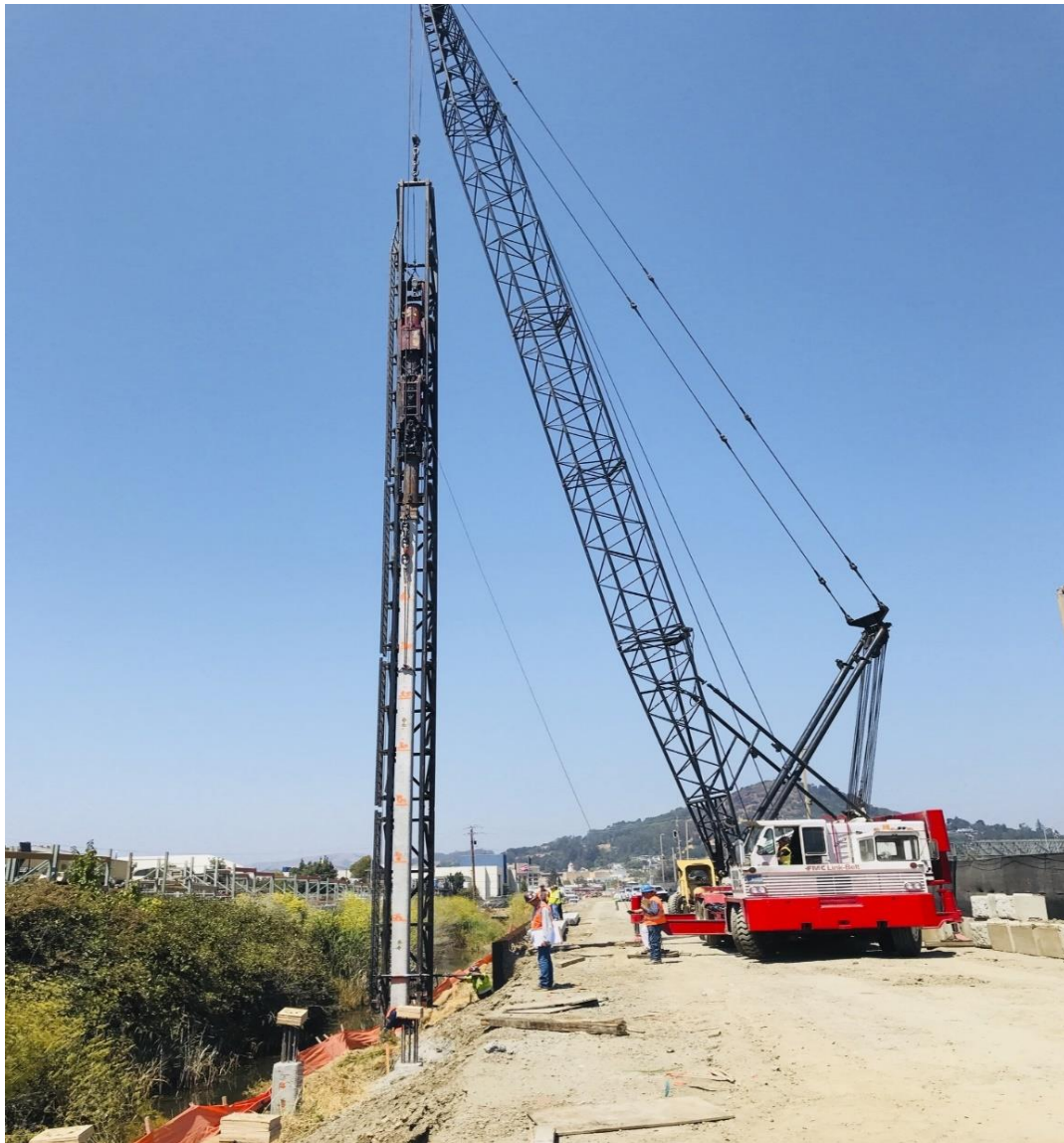
Multi Use Pathway, Sheet Pile Driving
