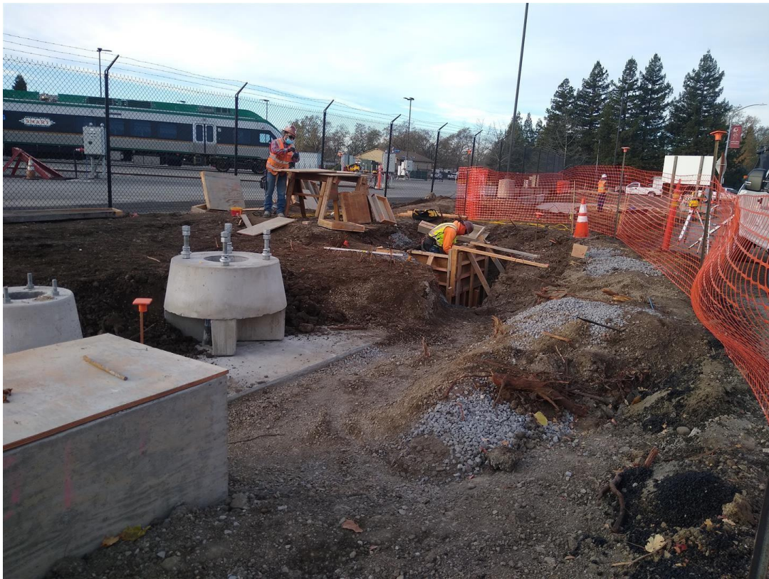
Constructing Traffic Signal and Grade Crossing Gate Pole Foundations – Airport Blvd, Santa Rosa
