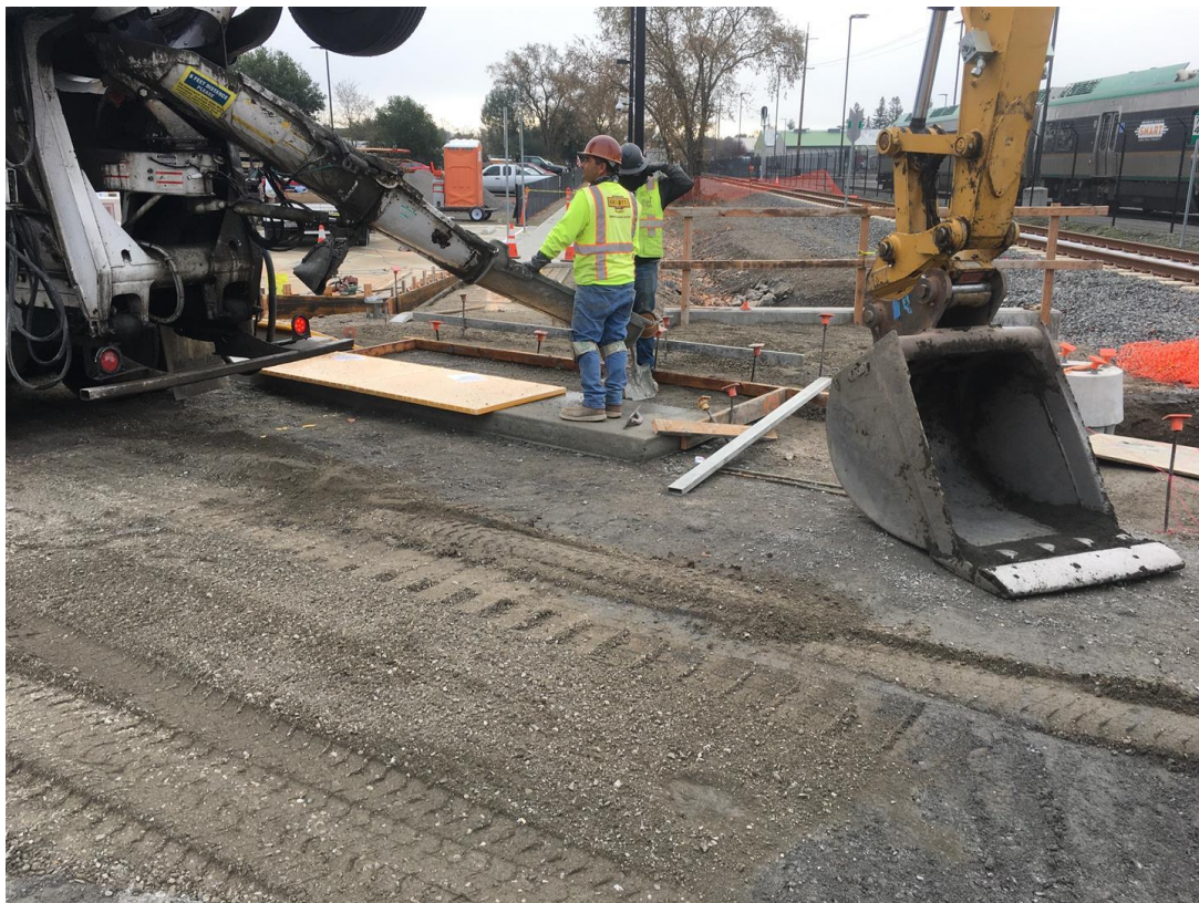
Pouring New Curb and Gutter – Airport Blvd, Santa Rosa
