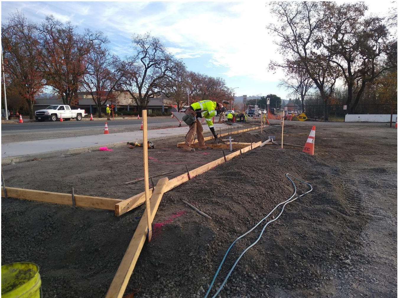
Framing Area for New Sidewalk and Bus Stop Area – Airport Blvd, Santa Rosa
