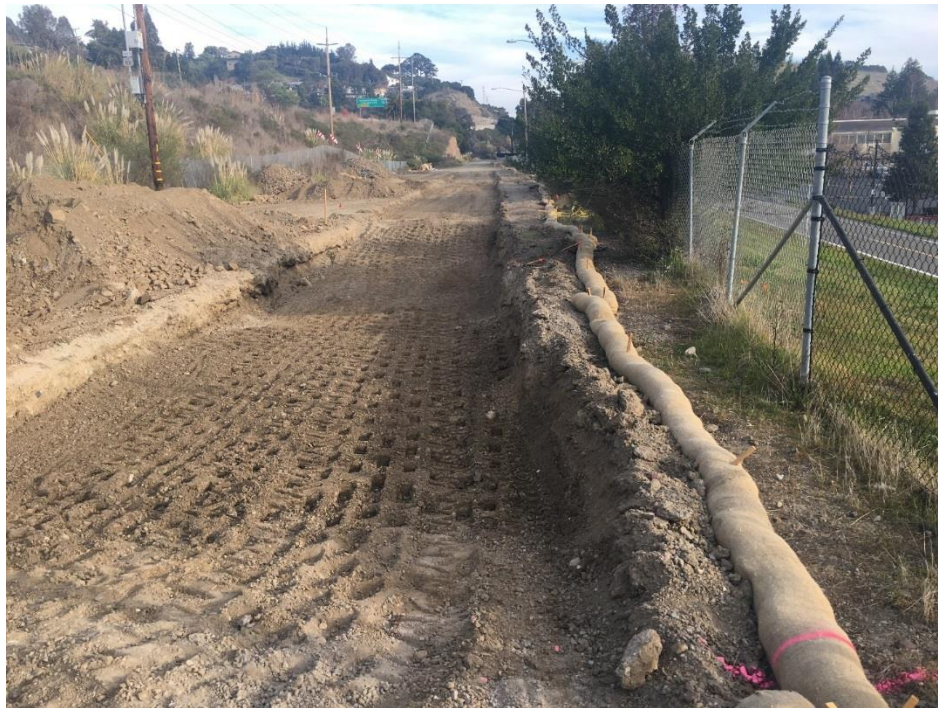
The crews have removed ties and backfilled at the site of the Larkspur Station foundation.
