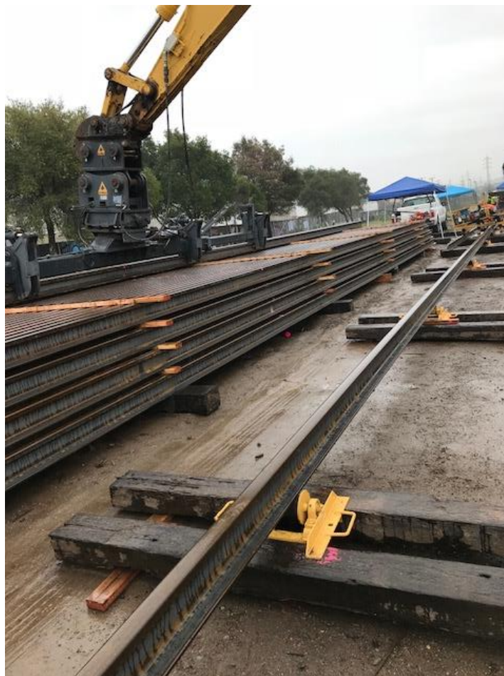
The rail is being prepared for welding from Andersen Drive to Unnamed Channel.
