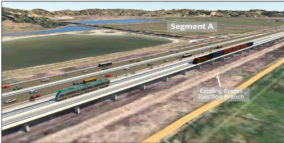
Figure 11. SR 37 Segment A View with Freight Looking Northeast
