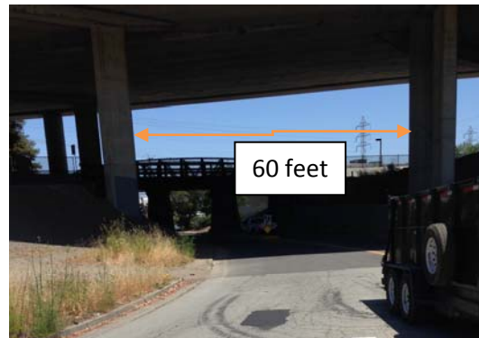
Figure 11 – Highway Support Width
