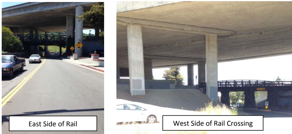
Figure 9 – Auburn Street Structural Photos
