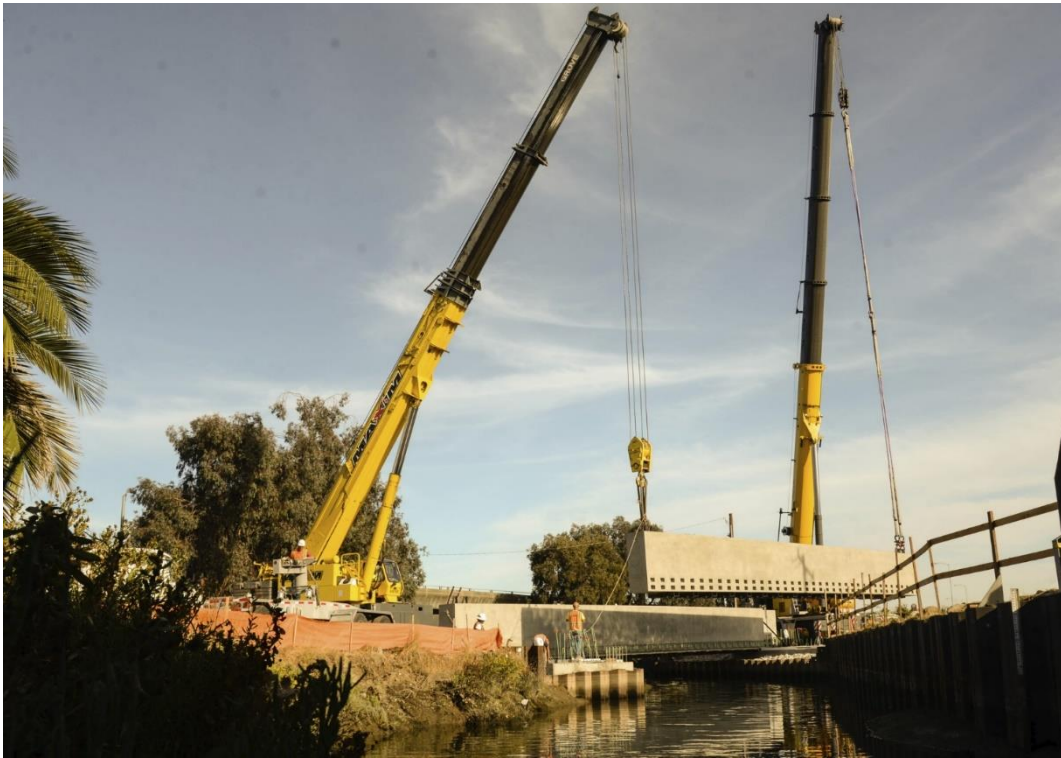
San Rafael Creek Bridges – installation of precast bridge girders
