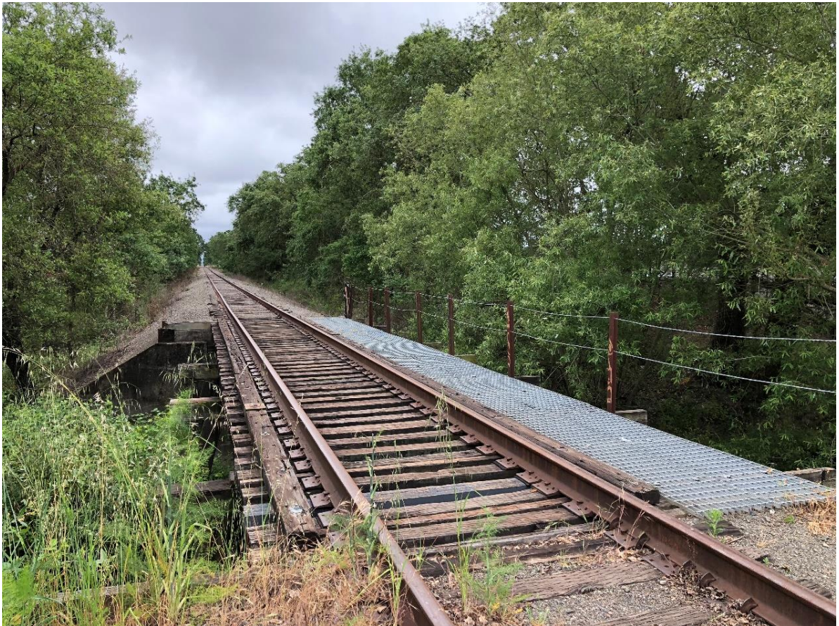
Existing Timber Trestle along the Windsor Alignment
