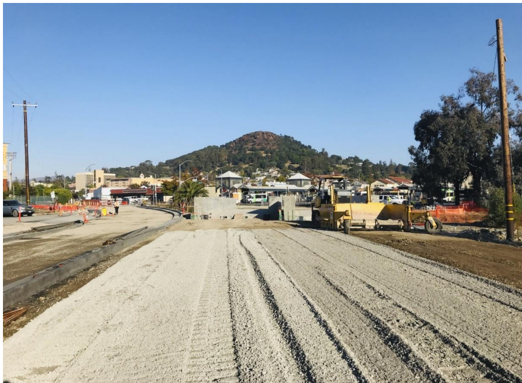
Francisco Blvd West – preping track subgrade
