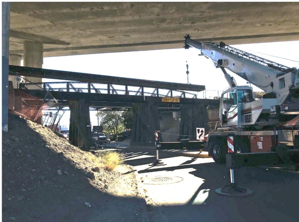
Auburn Bridge – installing new bridge beam
