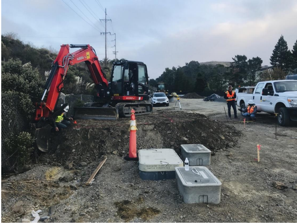
Signal house foundation construction at the Larkspur Station
