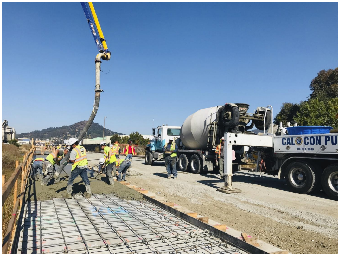
City of San Rafael Pathway – concrete topping slab
