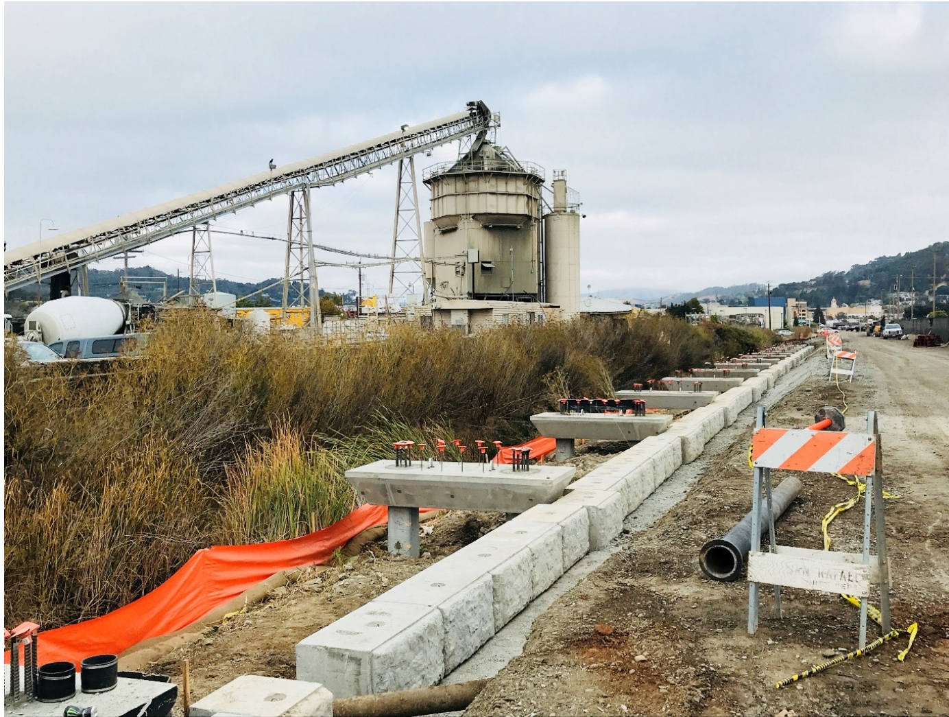
Andersen to Rice Pathway Construction (For the City of San Rafael)
